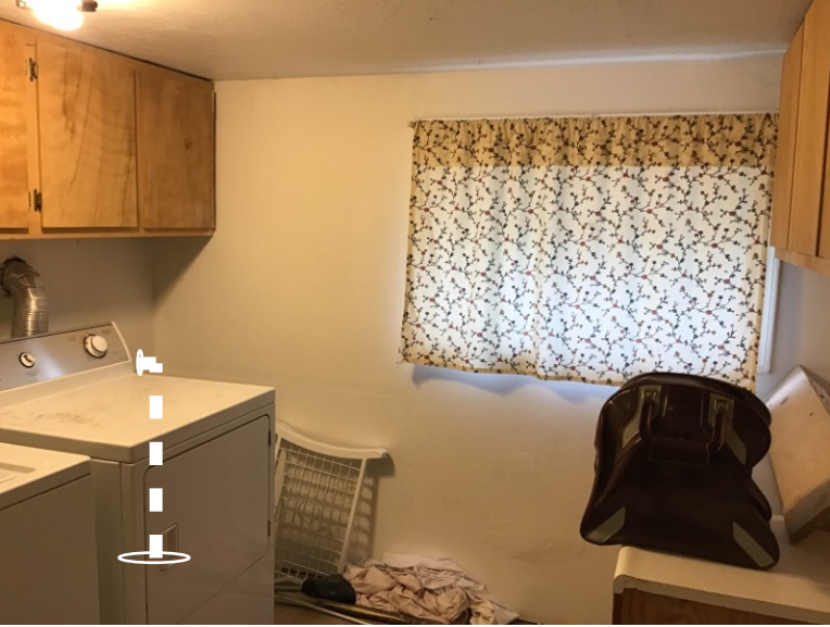
Suction point location in basement laundry room
