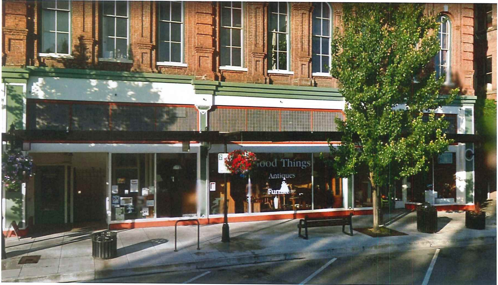
PHOTOGRAPH D Current Storefront Configuration
