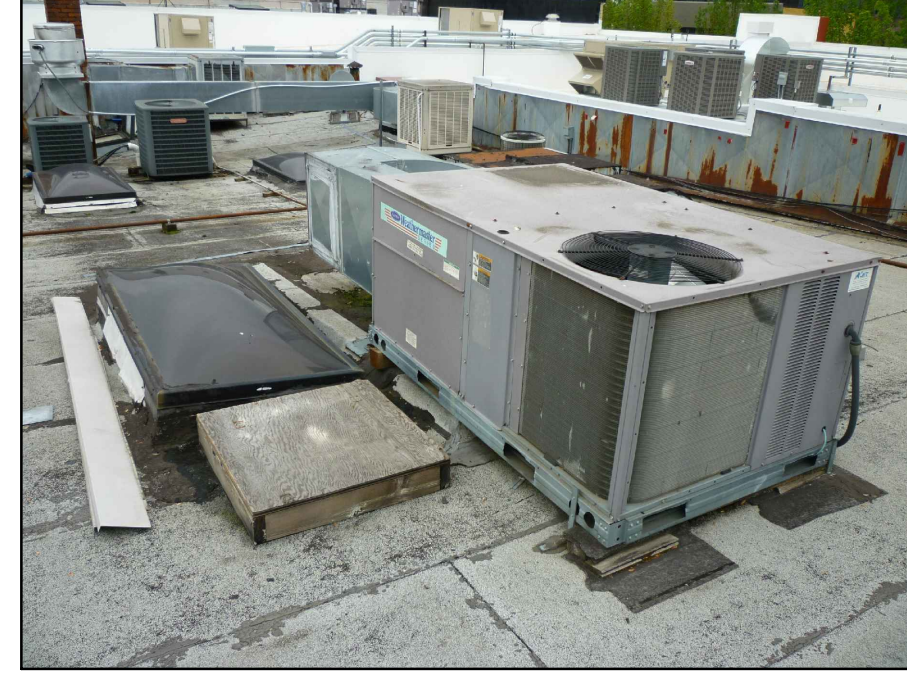
PHOTO OF EXISTING ROOF TOP HVAC UNIT TO BE REPLACED
