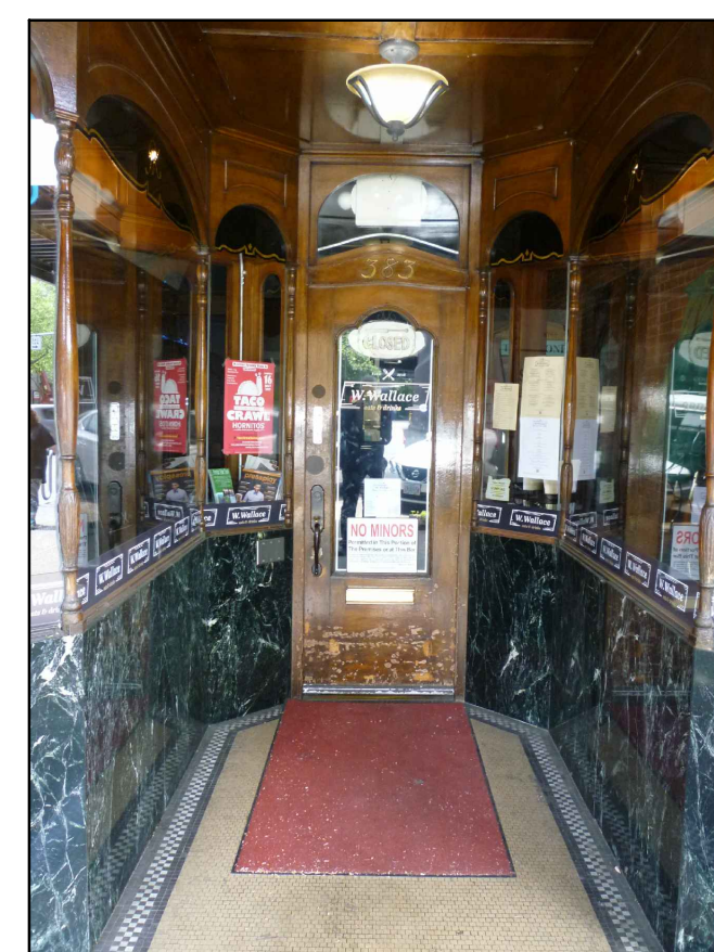
C. WALLACE ENTRANCE; EXISTING WOOD PANELING AND TRIM TO BE REFINISHED. LIGHT FIXTURE TO BE REMOVED AND REPLACED
