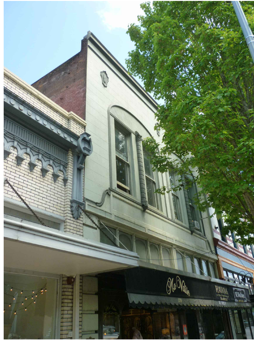
EXISTING SOUTH FACE
