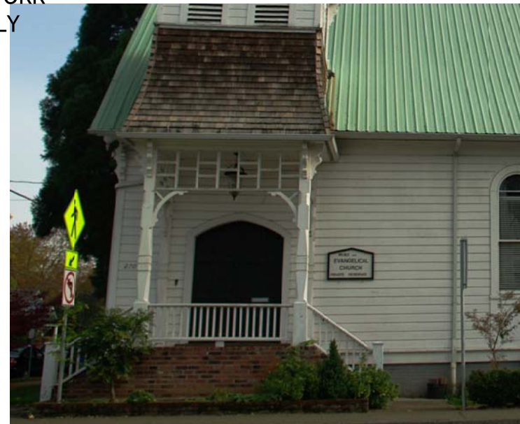
EXISTING HOUSE AND PORCH
