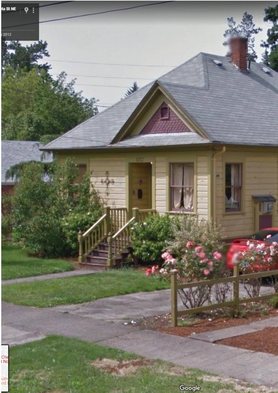
SHOWING PREVIOUS STAIRS NOW REMOVED DUE TO FAILING MATERIALS
