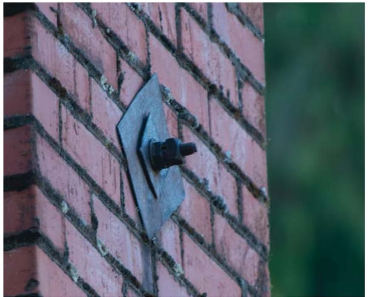
*Figure 22: Chimney Brace Plate Detail*
