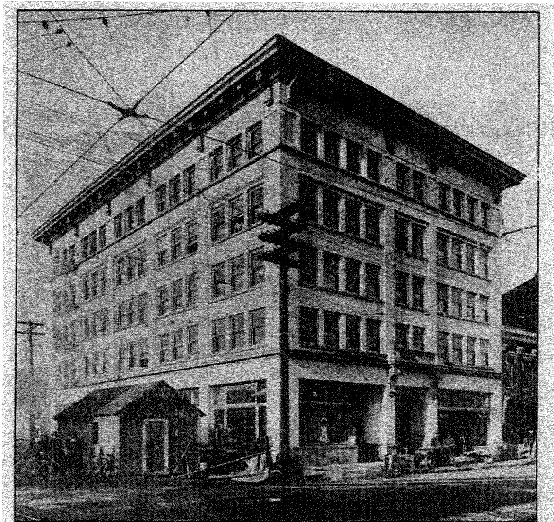
—P. A. Legg, Architect. New Five-Story Steel Frame Concrete and Pressed Brick Building of the United States National Bank just Being Completed.
