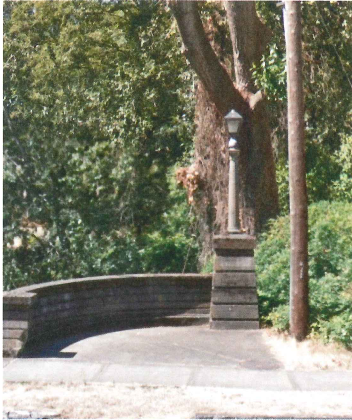
Northwest end of Church Street Bridge, Lighting Detail – (typical)
