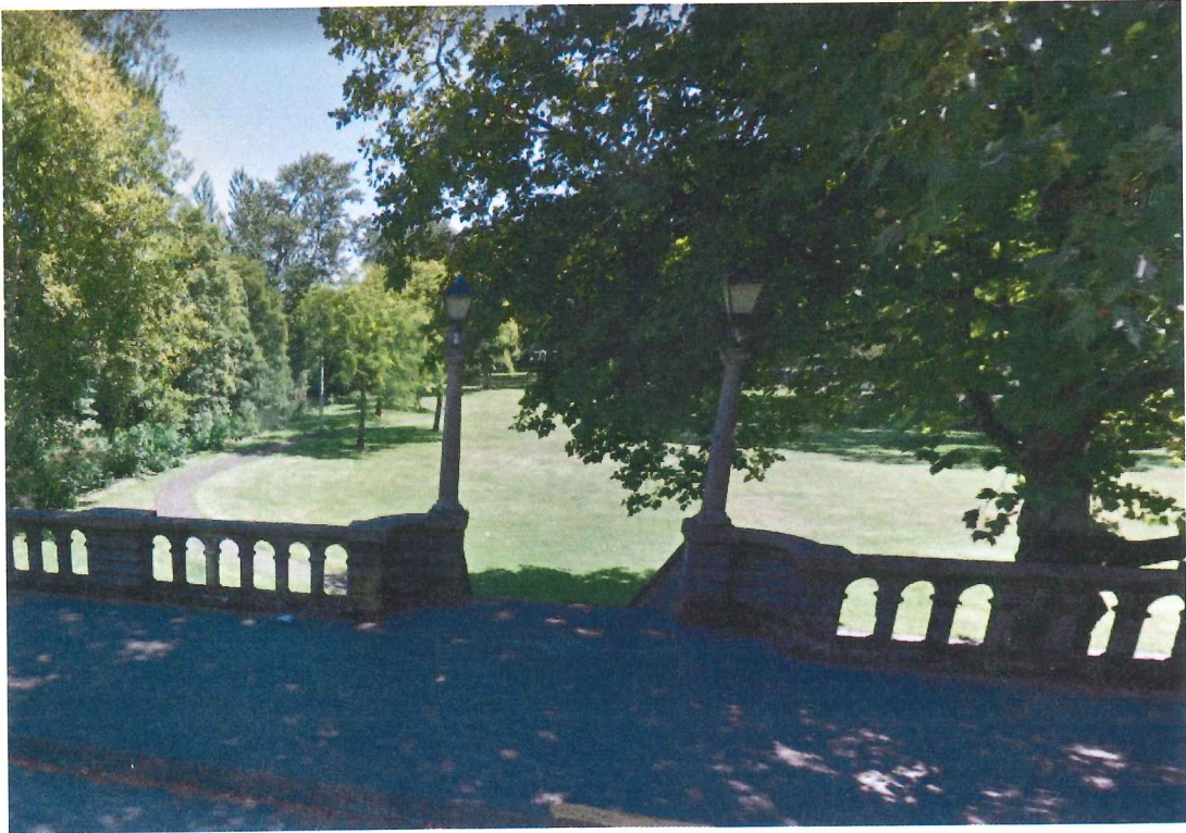
East Bridge Rail- Center, Church Street Bridge
