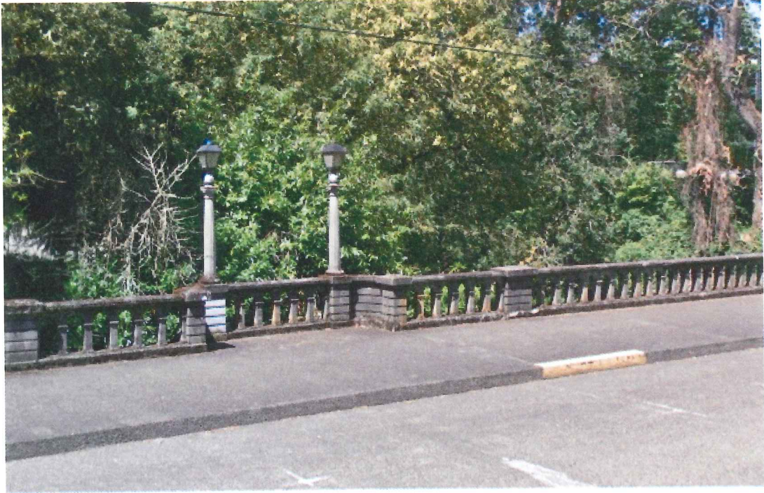
West Bridge Rail- Center, Church Street Bridge
