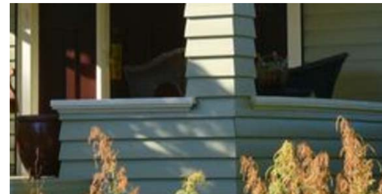
3 SEAT BOARD/WALL CAP TRIM NTS
