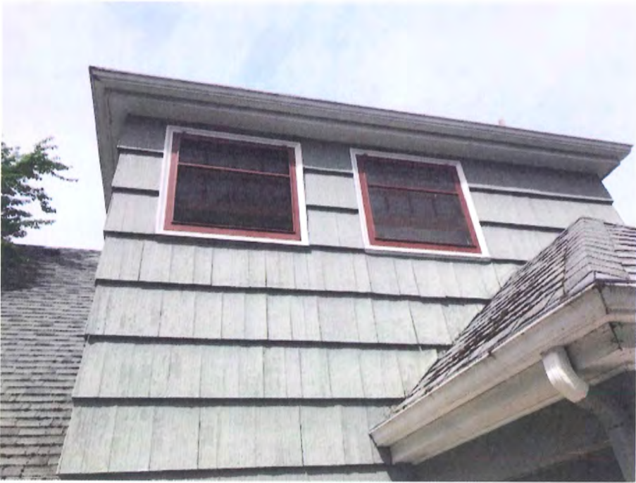
South Façade – 2 nd Floor – Window 10, 11, historic
