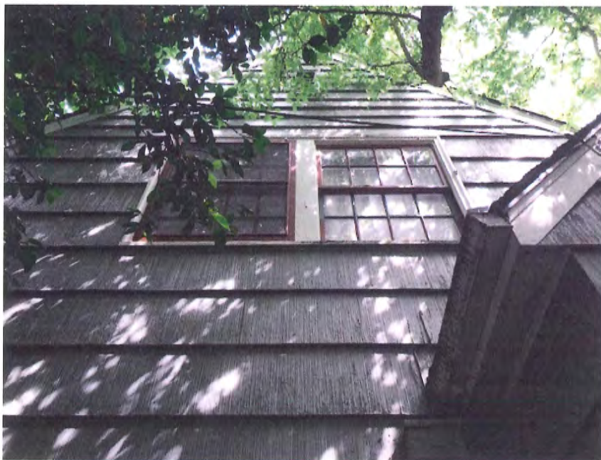
West Façade- Second floor – Windows 13, 14
