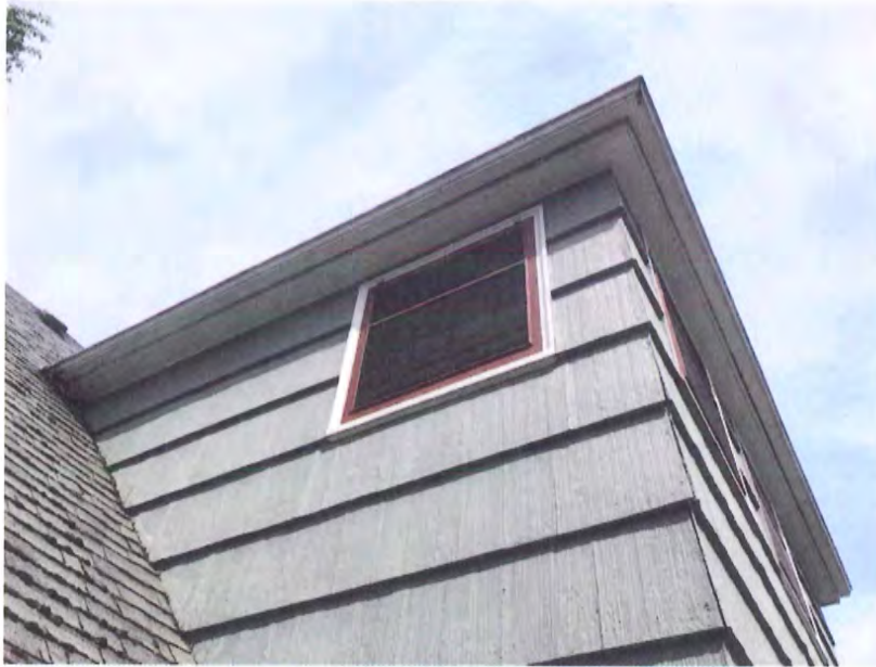
Southwest Façade – 2 nd Floor – Window 12, historic
