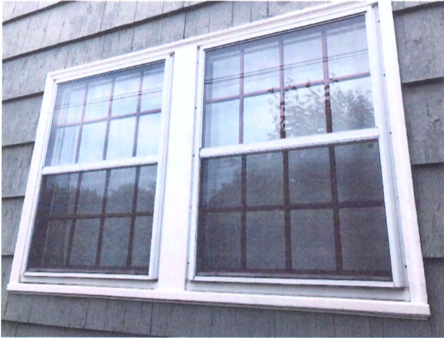
East Façade – 1 st Floor- Window #1, 2
