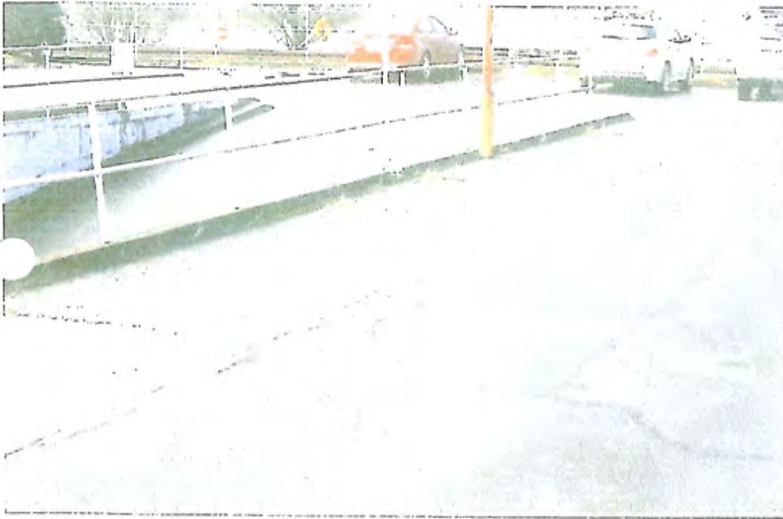
14. "Guardrail" at Ramp
