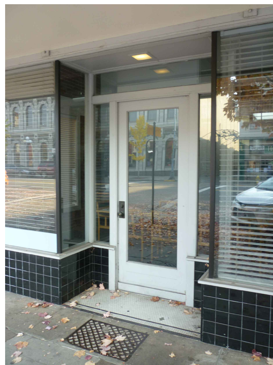
PHOTO 1 - EXISTING SINGLE DOOR
