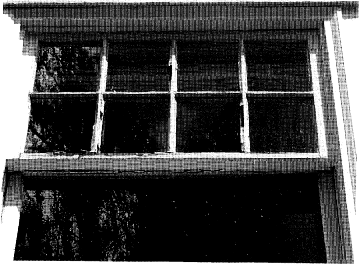
Window (typical) in Poor Condition
