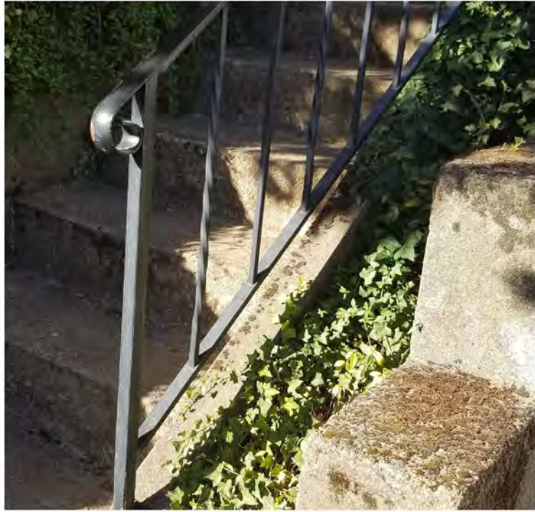
1 EXISTING HANDRAIL (PHOTO) SCALE:
