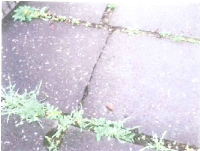
Cracked paver
