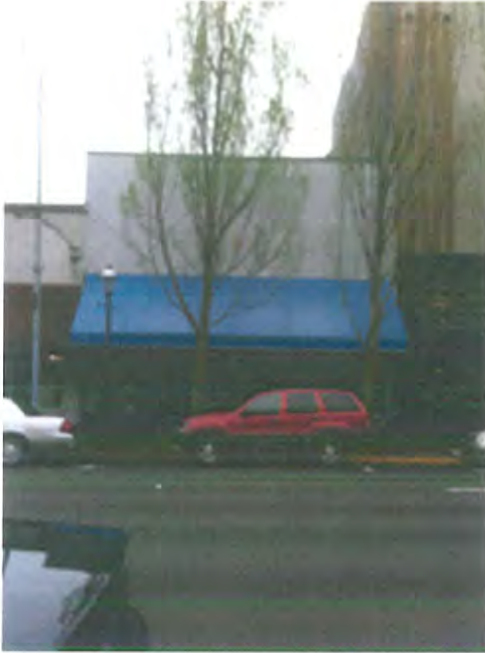
PHOTO OF OLD AWNING JUST PRIOR TO REMOVAL OF AWNING DONE IN 2012.
