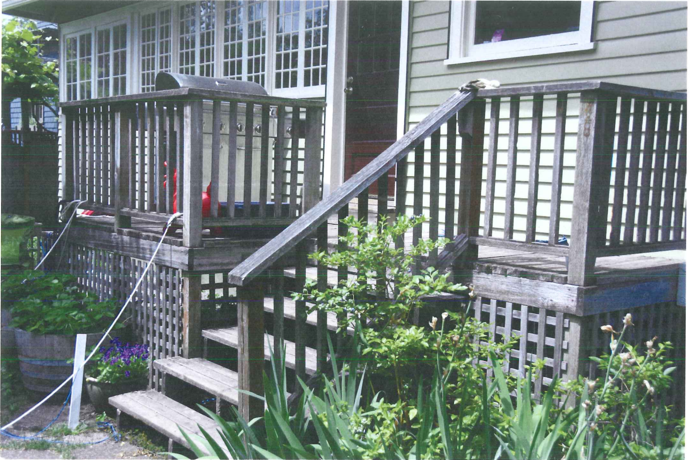
Existing deck structure
