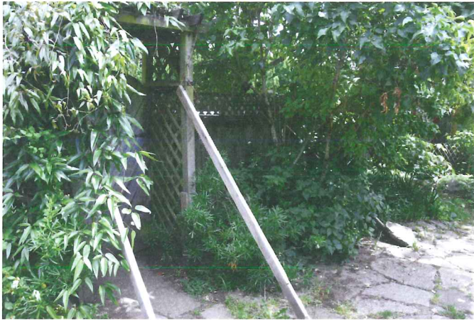
Supports on house side of fence
