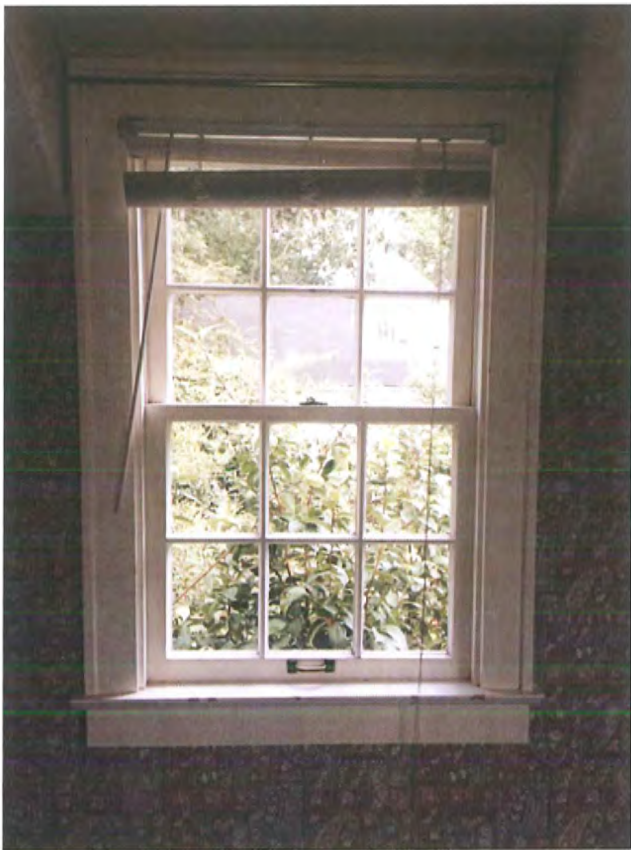
Northwest window, caretaker bedroom
