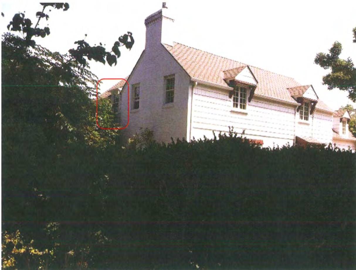
Northwest window, view from right-of-way
