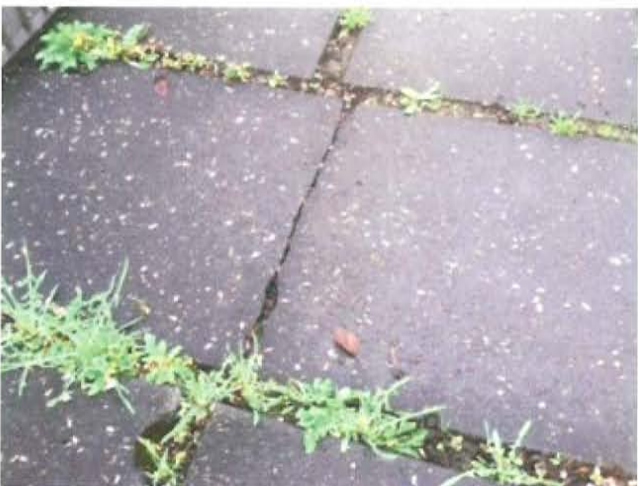
Cracked paver
