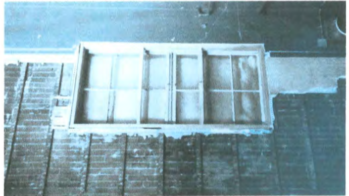
Interior window West wall (south of corner)
