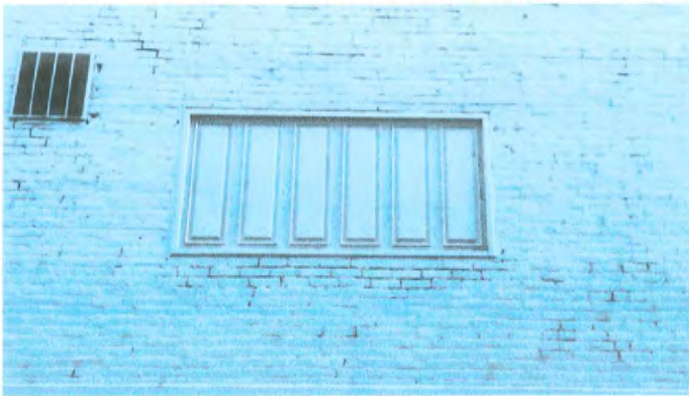
Exterior West wall (south of corner)
