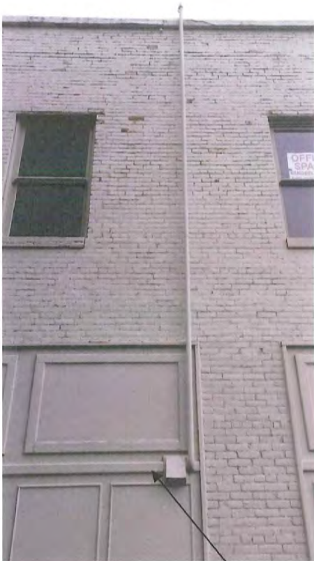
Existing venting Proposed: one additional vent to match
