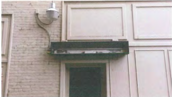
Existing sign on west Wall 1' x 6'
