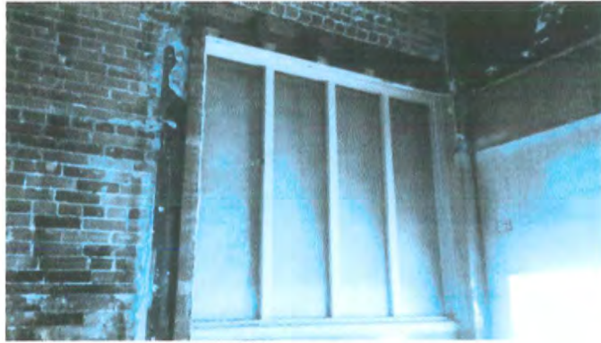
North West Interior (corner window)
