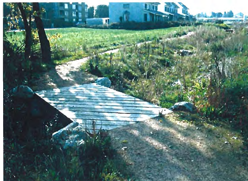
Pedestrian path crossing a green drainage corridor
