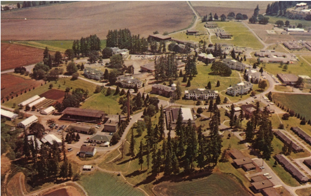
Aerial view of Fairview Training Center from the northwest.
