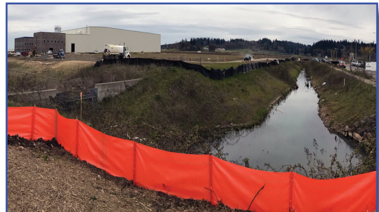
Henningsen Cold Storage second location at Mill Creek Corporate Center.
