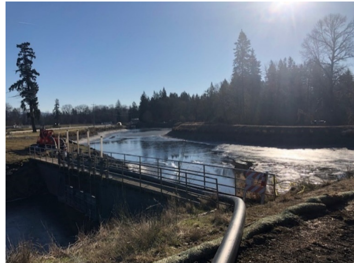
Geren Island water distribution system improvements
